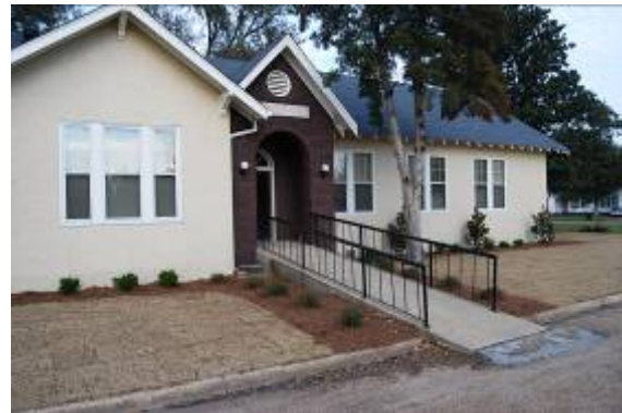
Refurbished Community House
